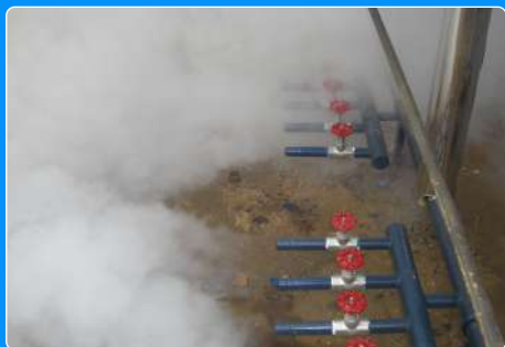
Portable boiler for site steam curing
