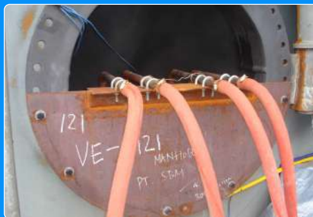
Install steam into vessel
