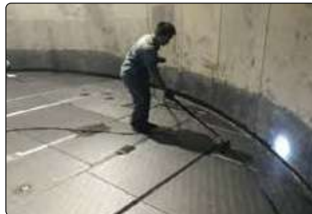
Inspection before Exhausting curing
