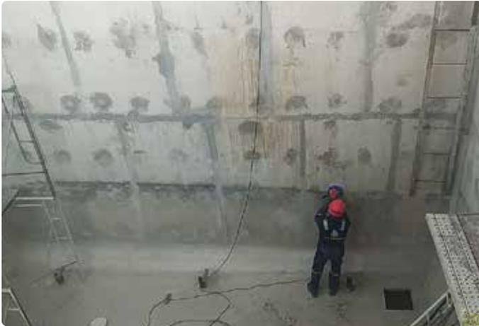
Surface preparation before apply primer coat PR-90
