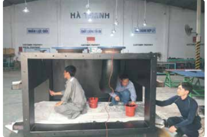
Lining butyl rubber on mining tank for anti-shock
