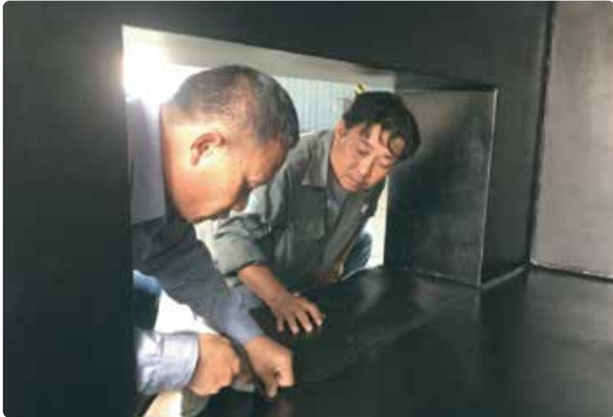
Lining square tank
