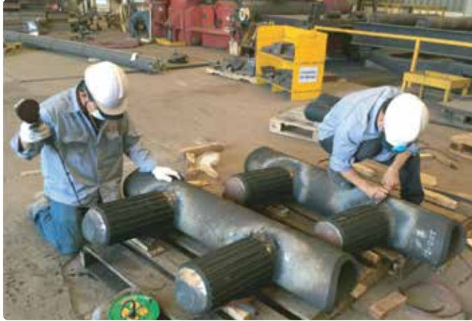
Finishing Neoprene Rubber lining for wind tower
