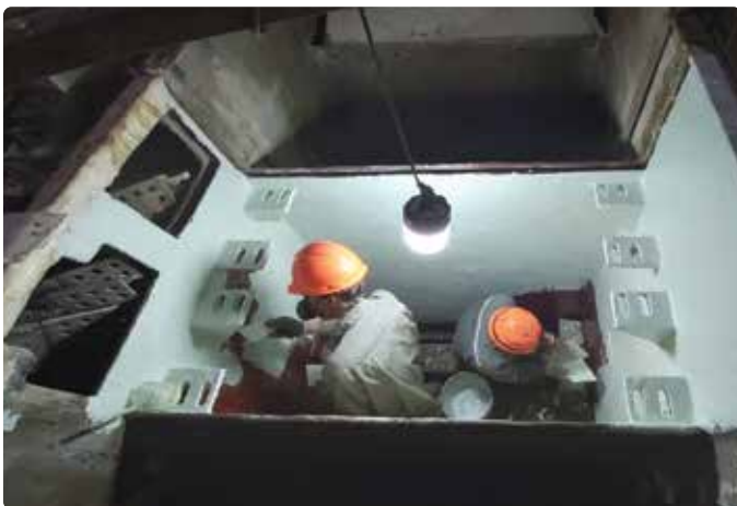
Pickling Resin Tank
