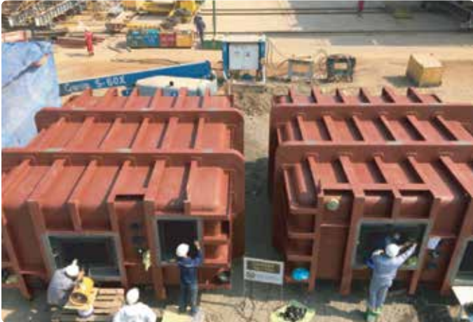
HCL tank on site lining
