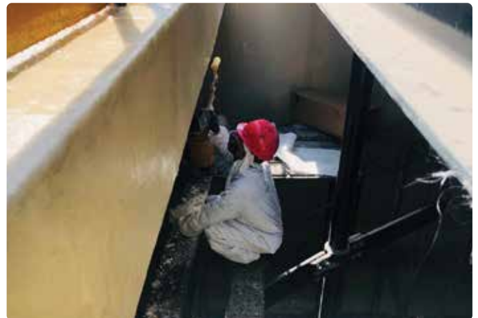
Lining FRP layer (M+M+SM) onto HF-161 layer
