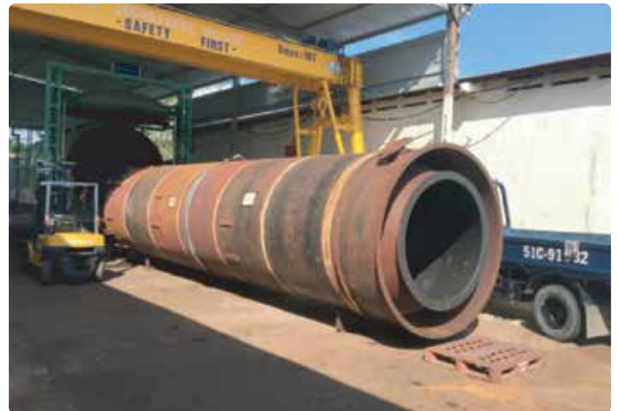
Lining hard rubber on chemical tower with over 10m length
