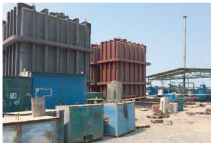
HCL tank on site lining for tanker
