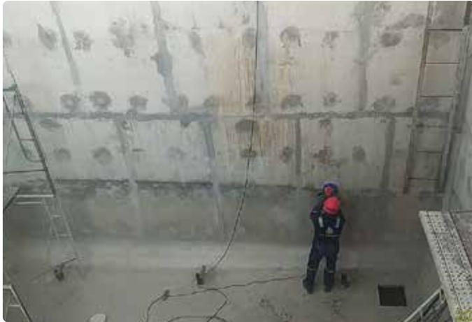
Surface preparation before apply primer coat PR-90
