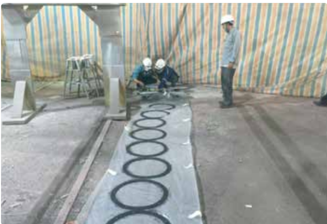
Cold lining EPDM gasket at site
