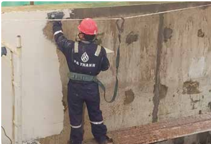
Apply OHJI HF-161 Flake lining by trowel
