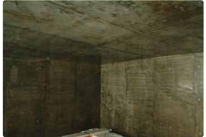
Completed primer coat PR-90
