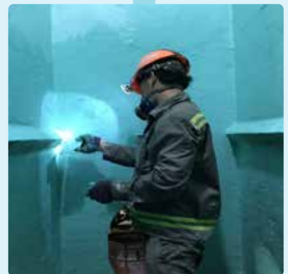
(3) 1st Coat of lining
