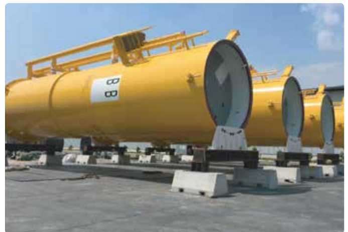
Neoprene-lined rubber completed on wind tower
