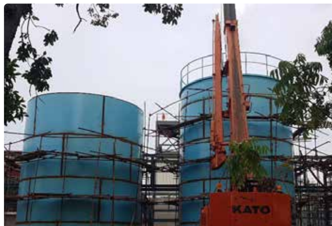
HCl storage tank on site lining
