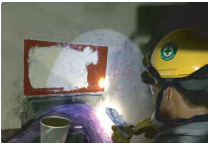
Flake lining spot repair
