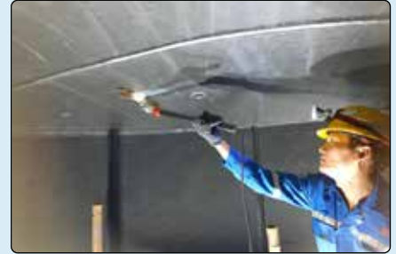
Ceiling pinhole check
