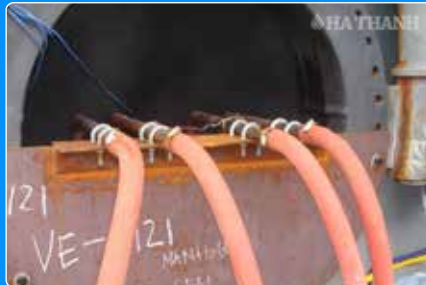
Install steam into vessel
