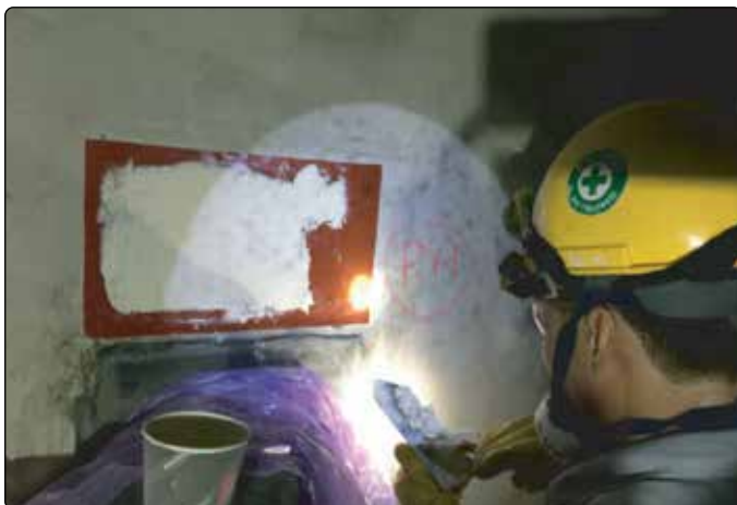
Flake lining spot repair
