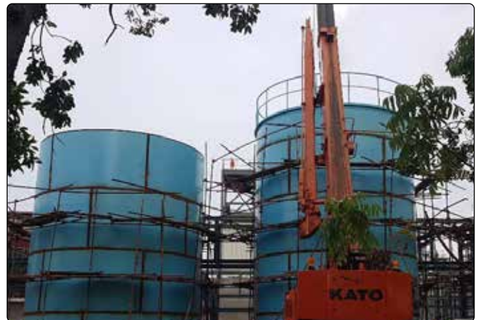
HCl storage tank on site lining
