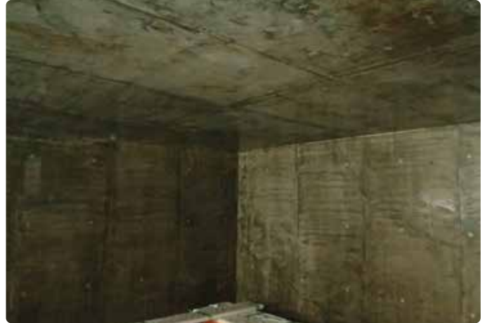
Completed primer coat PR-90
