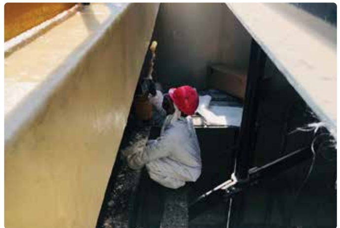
Lining FRP layer (M+M+SM) onto HF-161 layer
