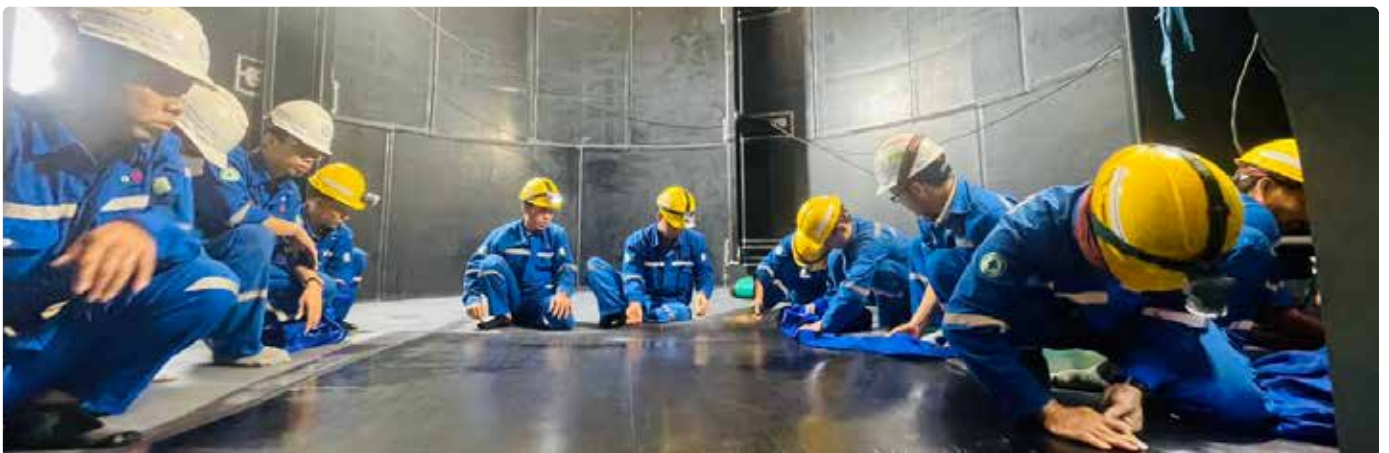
Ha Thanh team apply self cure rubber on slurry tank at site.
