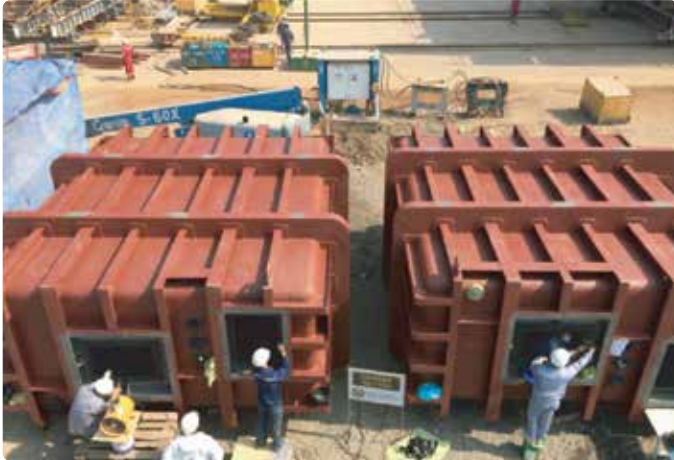
HCL tank on site lining
