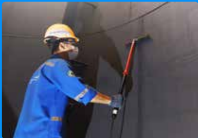
Pinhole inspection
