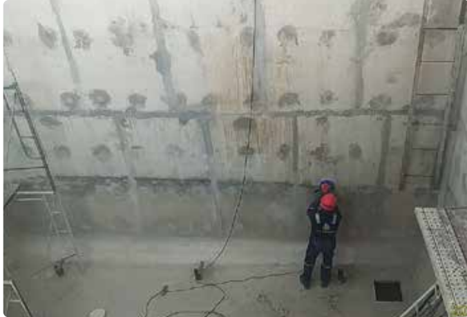
Surface preparation before apply primer coat PR-90
