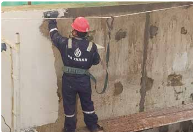
Apply OHJI HF-161 Flake lining by trowel
